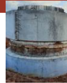
RETROFIT OF EXISTING FOUNDATIONS
