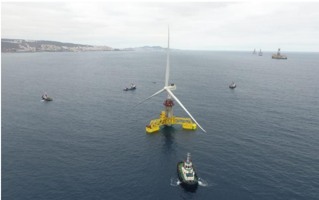
Installation: with low-cost means
