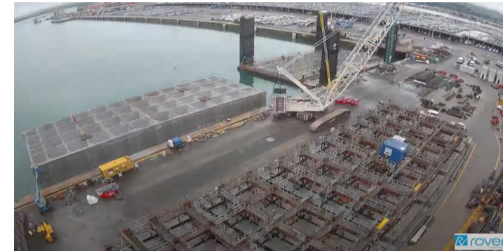
Concrete caissons construction in semisub barges
