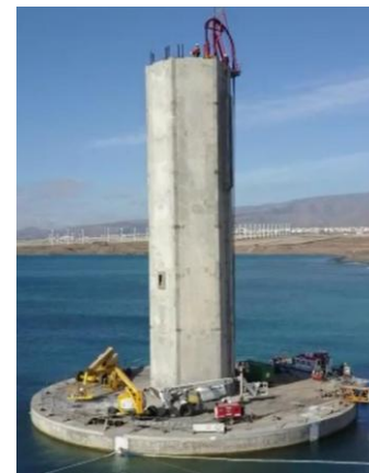
Base and first section of the tower (T0)
