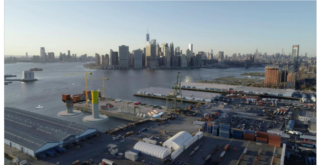
Caissons techniques for fabrication: floating docks and semi-submersible barges
