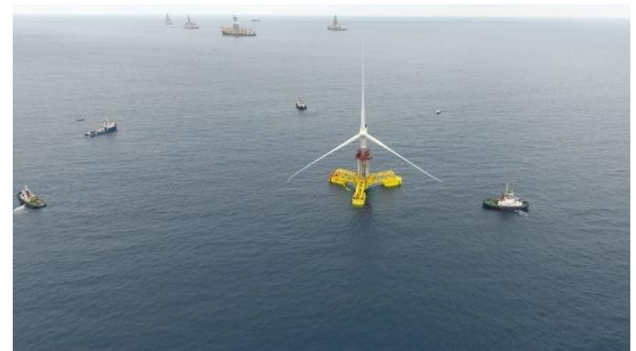
Configuration for ballasting onto the seabed (3 tugboats +1 control vessel)
