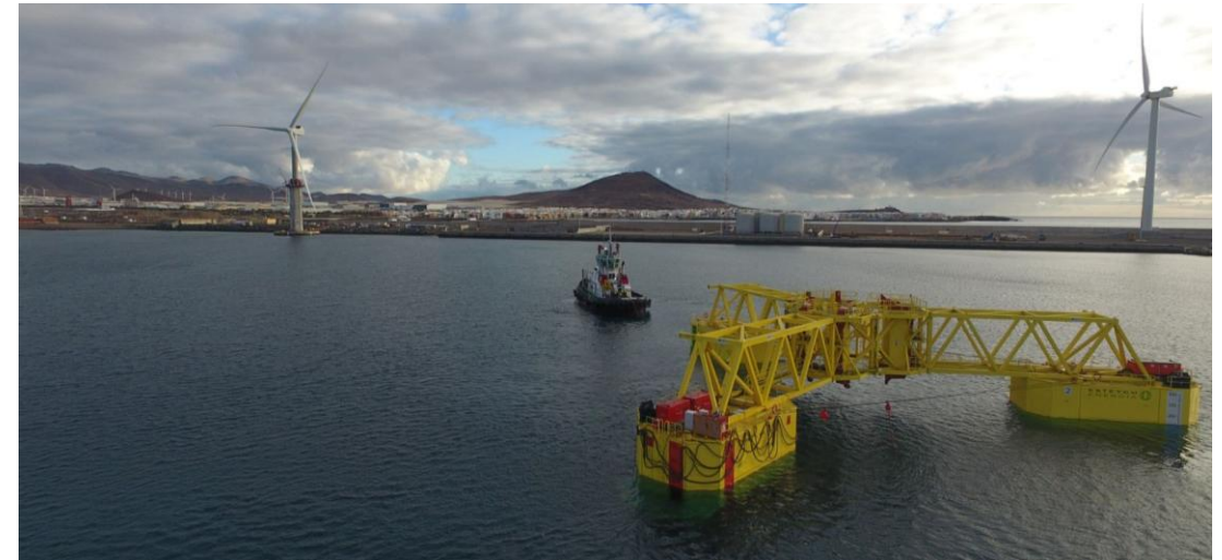
TIM approaching the ELISA GBS substructure
