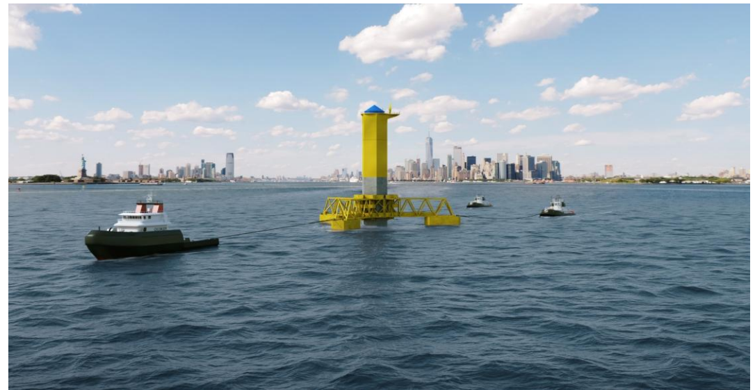
ELI GBS evolution with conventional independent installation of WTG with jack-ups
