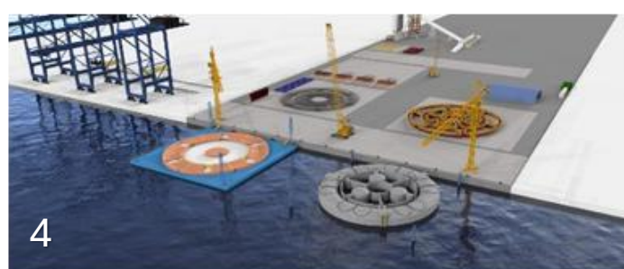
Example of construction sequence based on Airbarge technology for the concrete tanks of the WHEEL floater
