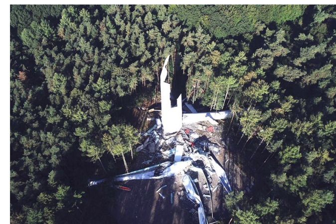
Hybrid tower collapse.
