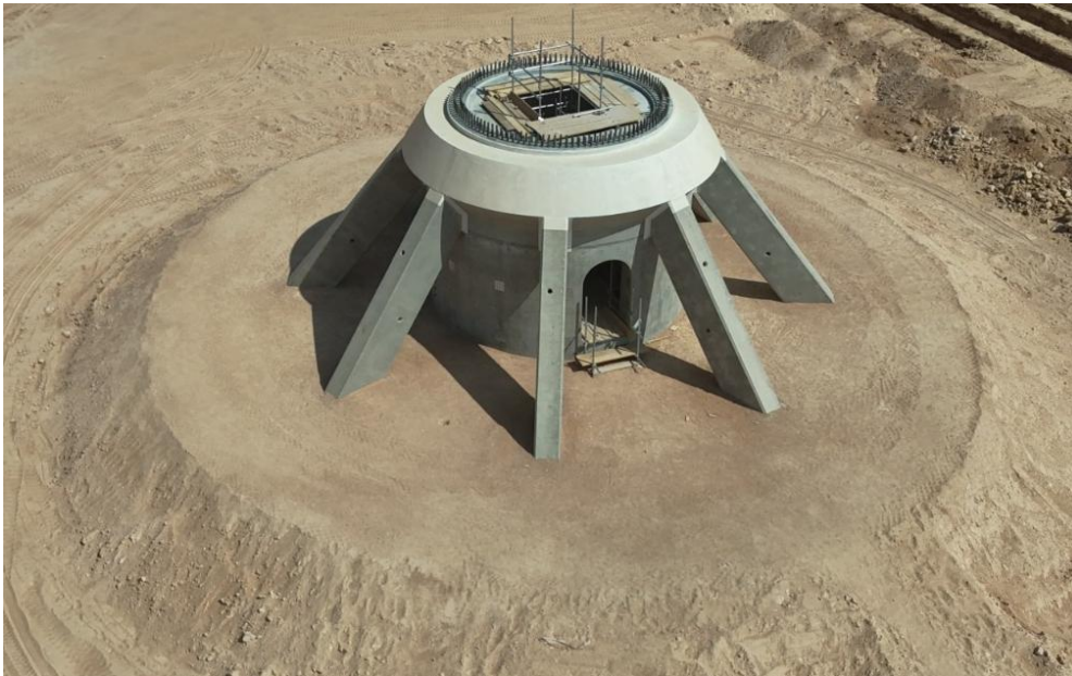
3. Upper flange construction, soil filling and turbine installation
