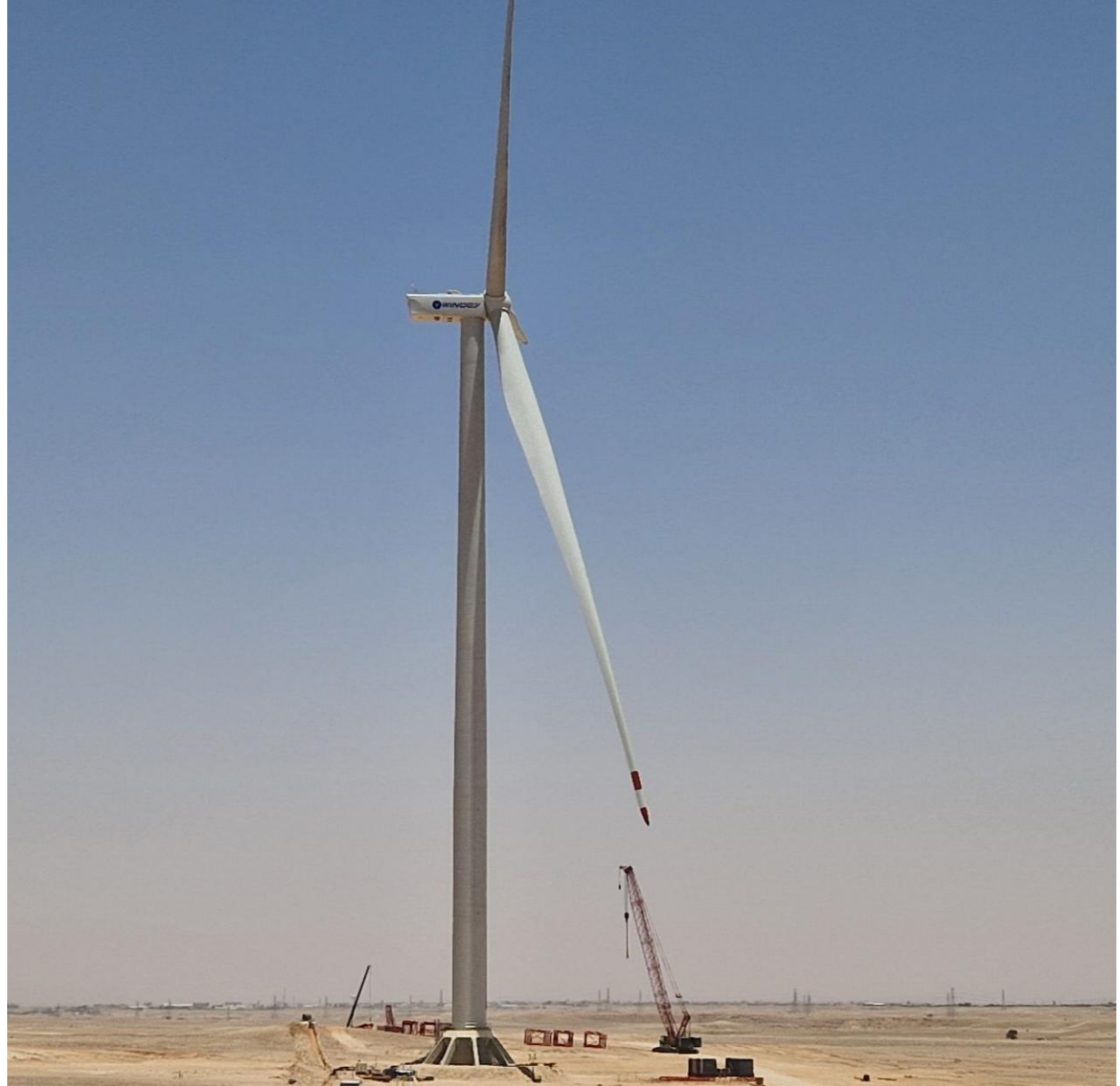
3. Upper flange construction, soil filling and turbine installation
