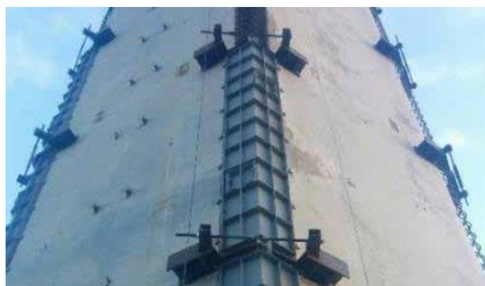
**Figure 20: External jacks on vertical joints**
