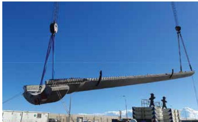
**Figure 19: Tilting of the panels**
