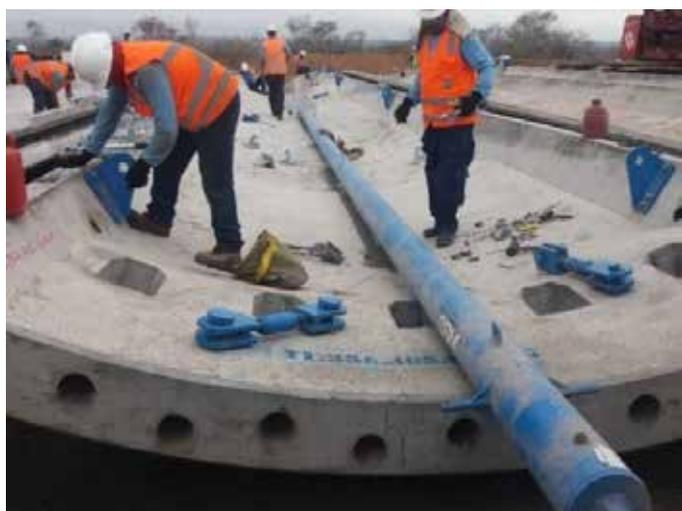
**Figure 17 and 18: Internal elements installation (working platform and prop on T4)**
