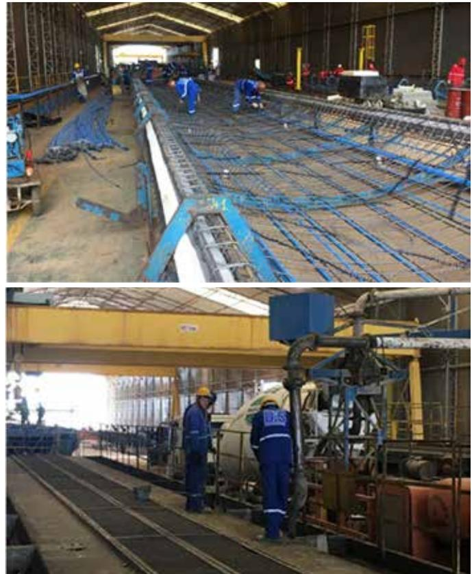
Figure 9 and 10: Reinforcement of the panels.
